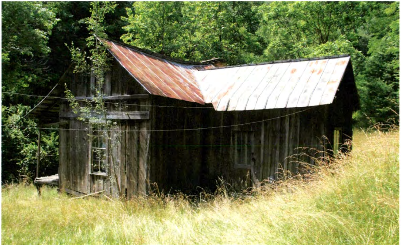
Boxed House, oblique rear view to south
