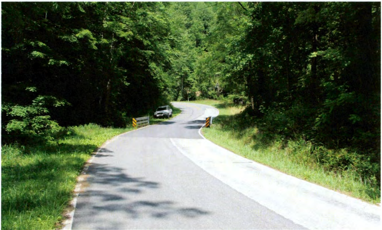
Bridge No. 121 on SR 1103 (Silvermine Road) over Silvermine Creek, view to northwest
