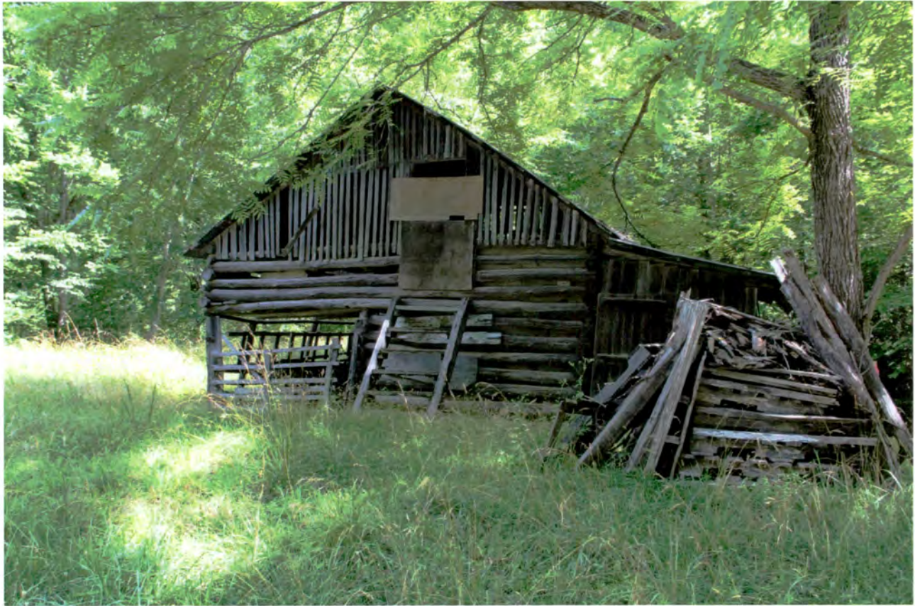
Log barn, view to north
