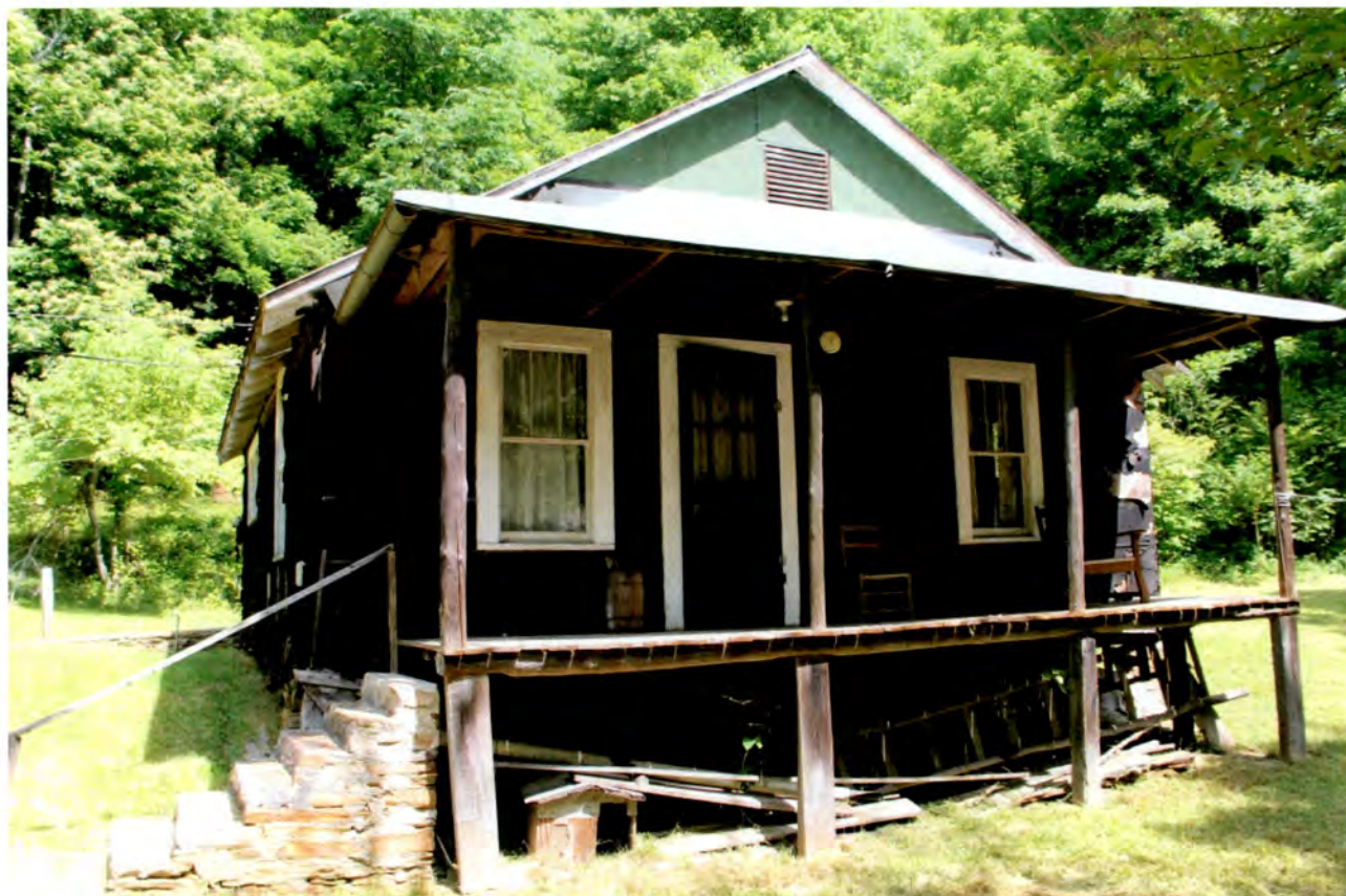
Truitt House, view to northwest
