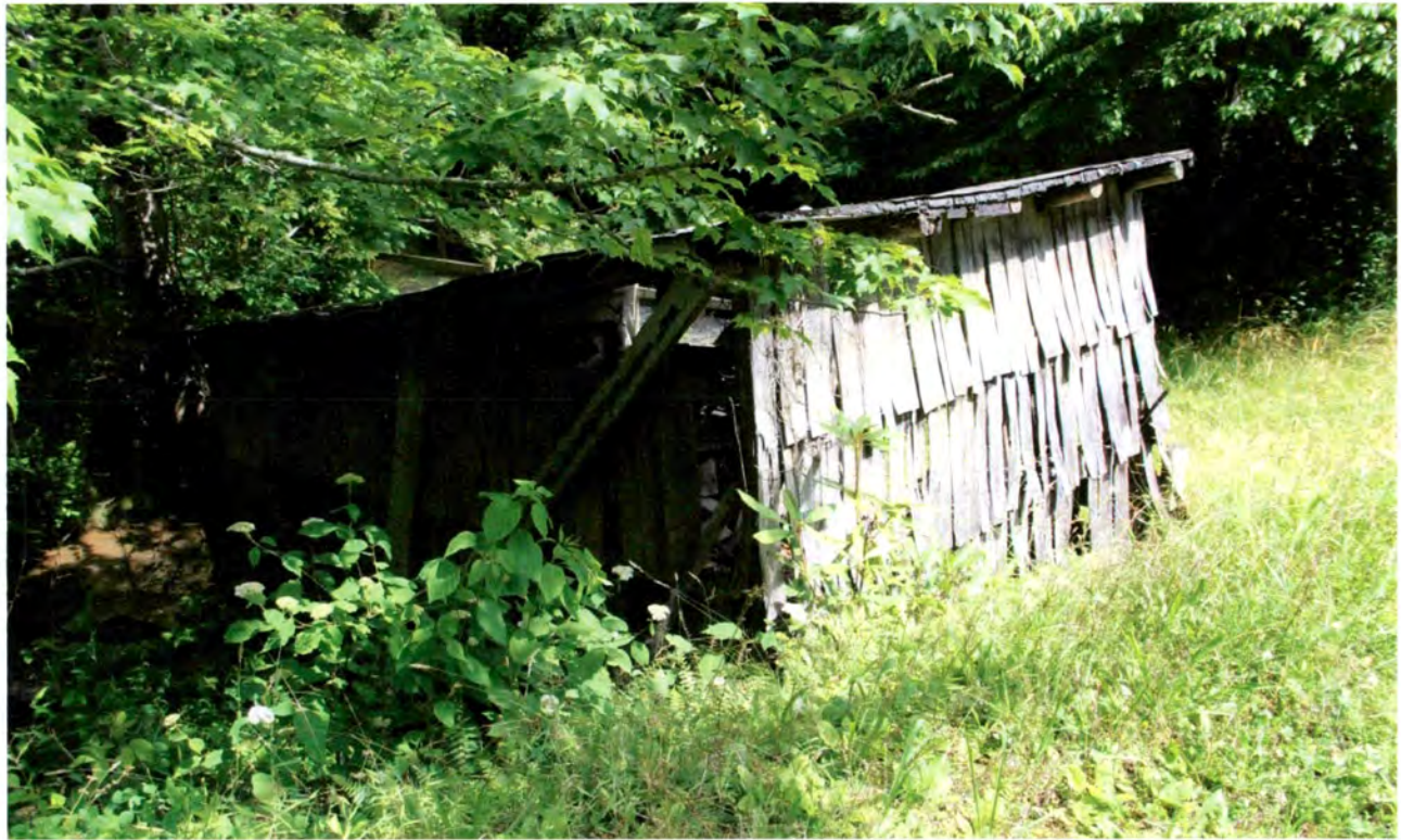
Wood shed, oblique view to north
