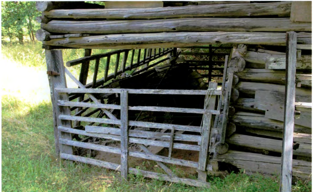
Log barn, detail, view to north
