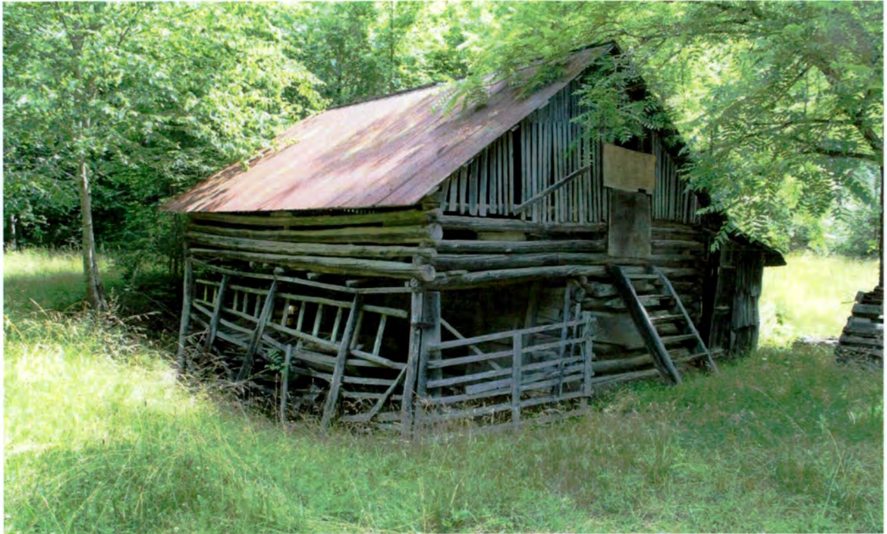
Log barn, oblique view to northeast
