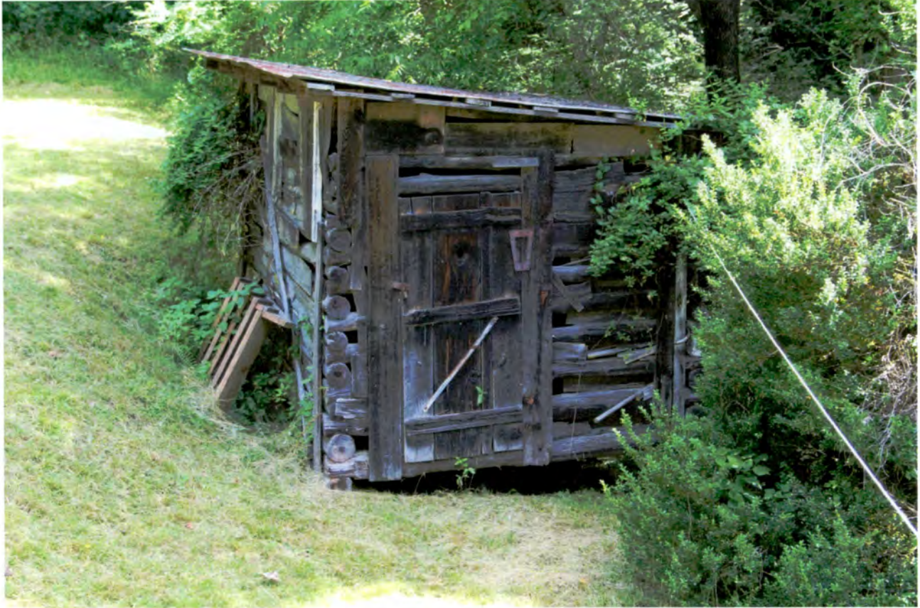
Crib, view to north
