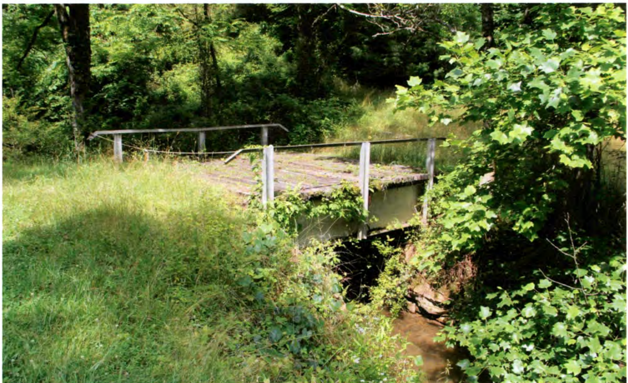
Vehicular bridge and access to property, view to southwest
