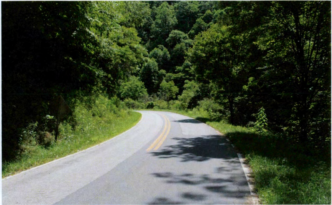
View to east along SR 1103 (Silvermine Road), east of Bridge No. 121
